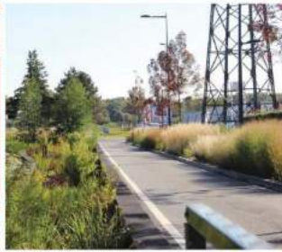
Swale buffer planted
